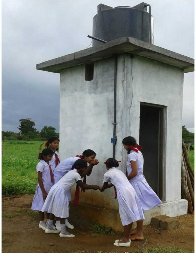
Water tank facilities to Mullikulam School Organised by RDO - DWF, with fund from Mr A. Agilan
